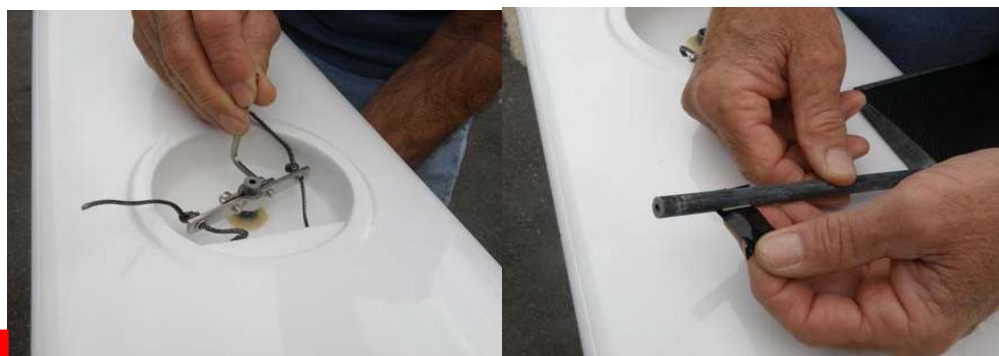
Photo 11. V-Series – loosen spreader bar assembly using allen wrench
